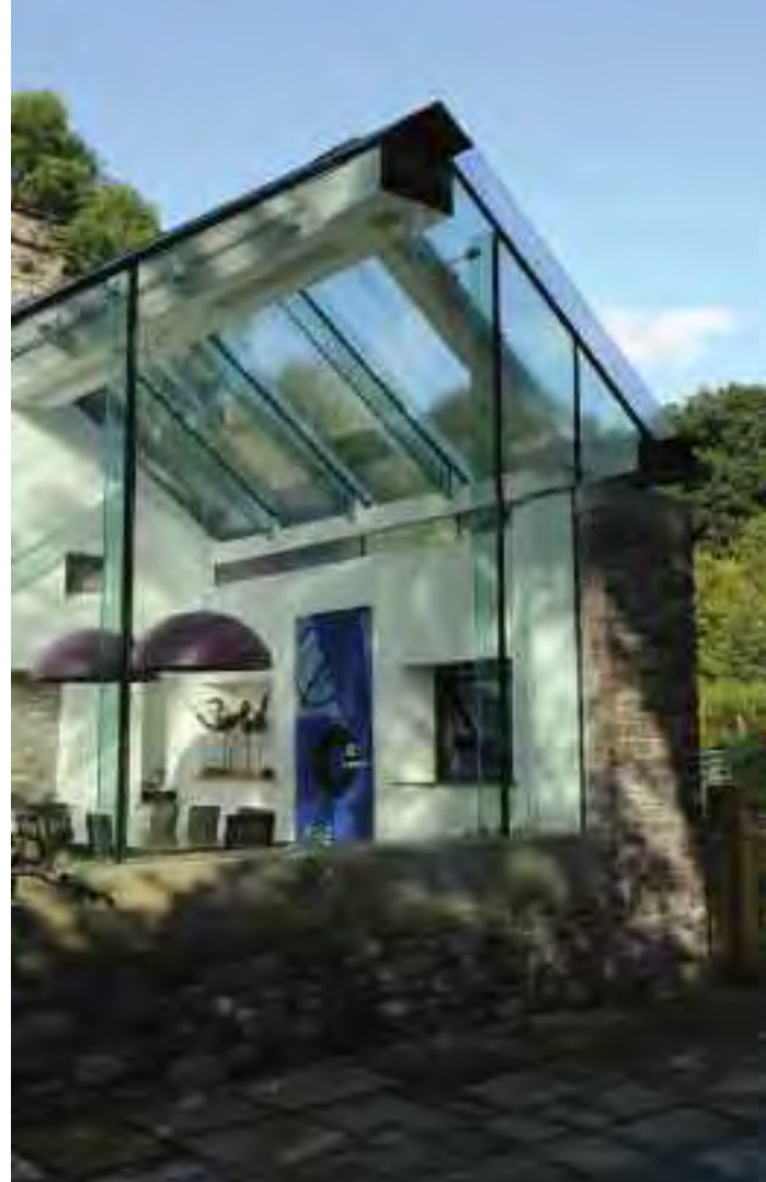
Farmhouse extension Builth Well Jeff Kahane & Associates
