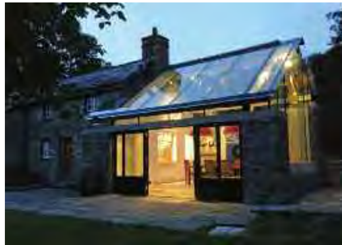
Farmhouse extension Builth Well Jeff Kahane & Associates
