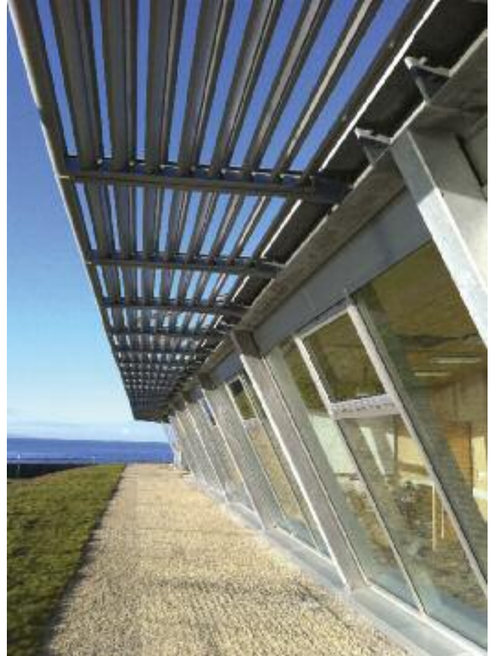
ACE 2 (Aberthaw Centre for Energy and Environment
