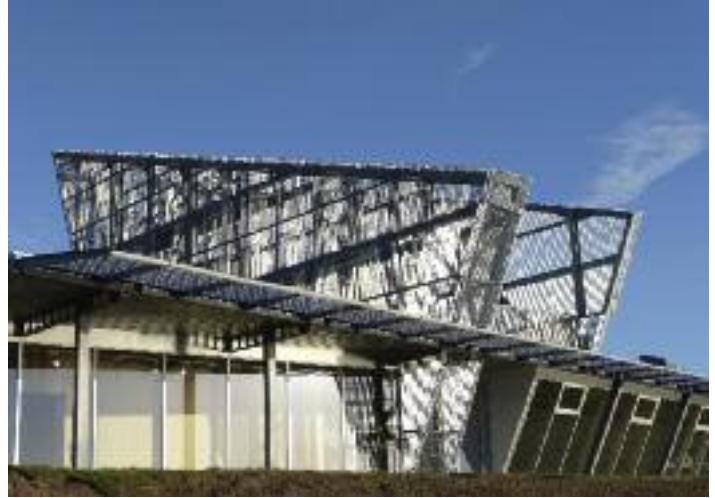
ACE 2 (Canolfan dros Ynni ac Amgylchedd Aberddawan) / ACE 2 (Aberthaw Centre for Energy and Environment)
